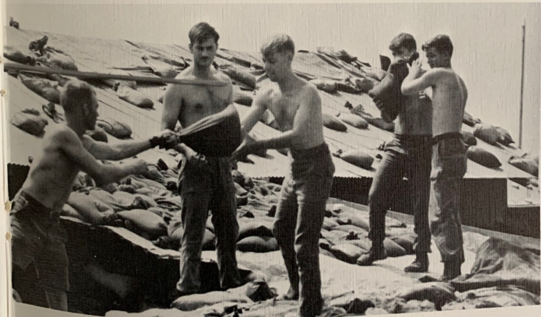
Bunkers and mortar pits rebuilt
